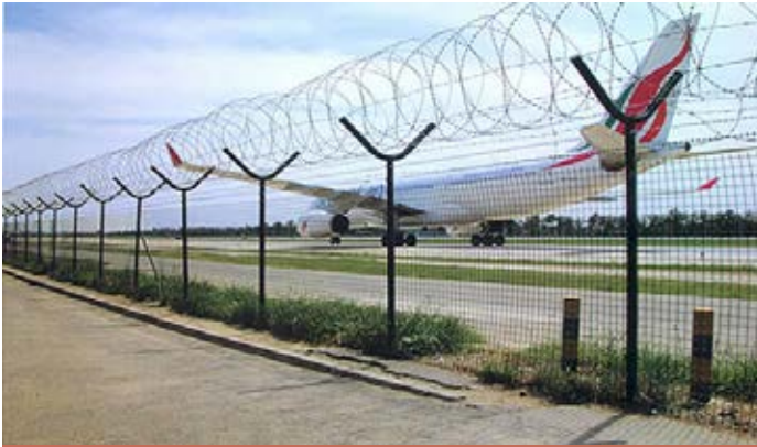
Well-maintained fence, at least 3m high, no gap at the bottom and dig protection are required
